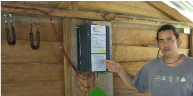
Generator sets and wiring system for electricity
